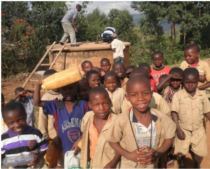
Waiting for the tank to be repaired
